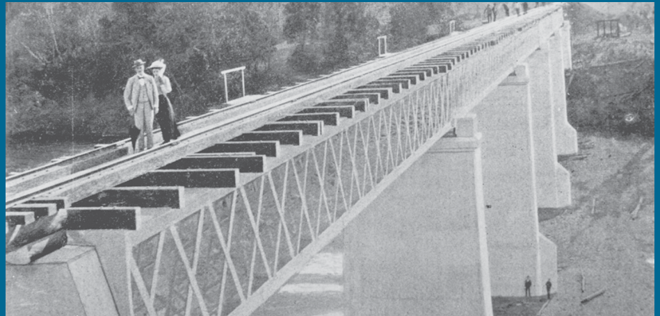
High-level railway bridge at Mirani, ca. 1897.
