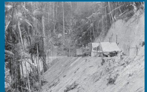
Construction of the road to Eungella, ca 1906-1907.
