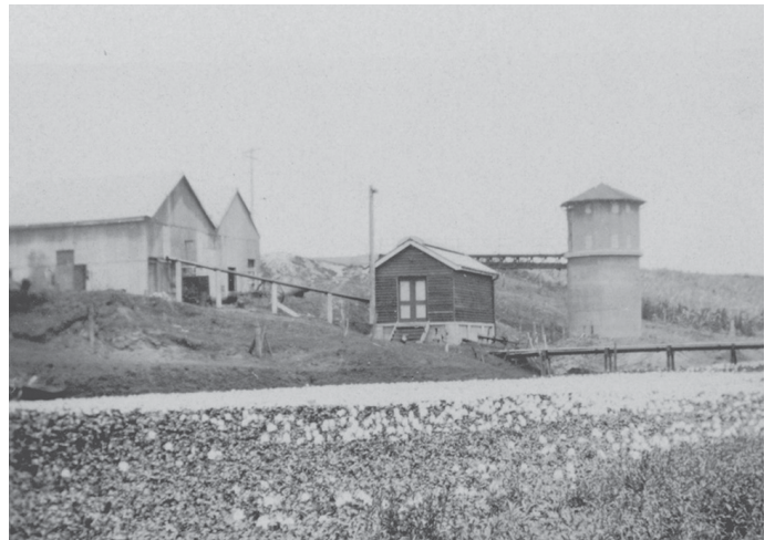
Mackay Water Plant, ca. 1910.
