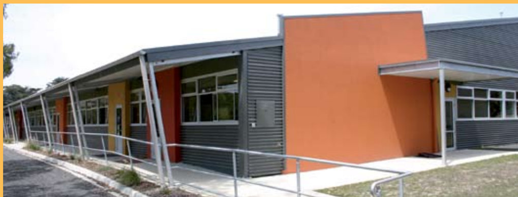
Below: The Technology Centre at St Ignatius College, Drysdale comprise workshops for wood and metal constructions and automotive and engineering practices.
