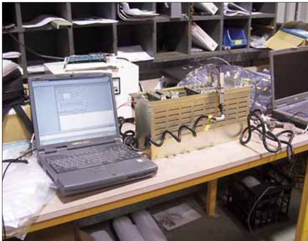
FIGURE 18: Power Car CPU Rack – Data Download
