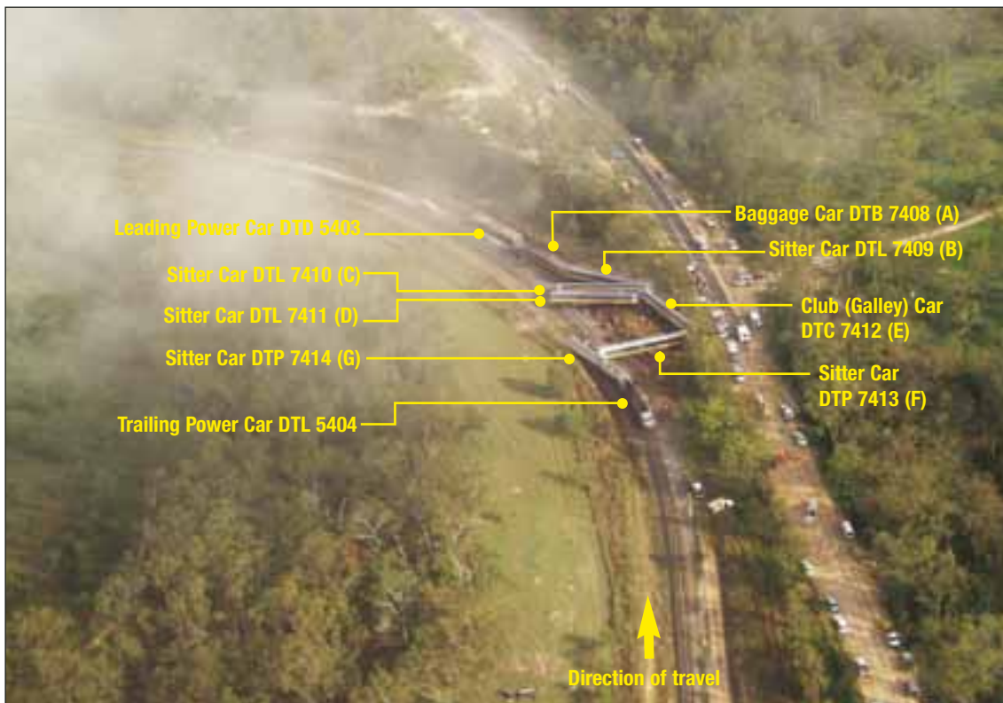
FIGURE 8: Aerial photograph of accident site, showing relative position of power car and trailer cars
