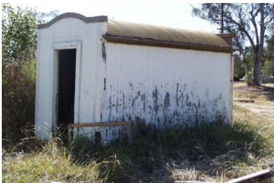
Corrugated steel clad shed, a surviving remnant of the 1911 Station complex.
