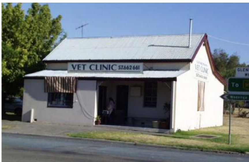
Former Post Office, (now veterinarian's clinic), 49 Beaconsfield Parade.
