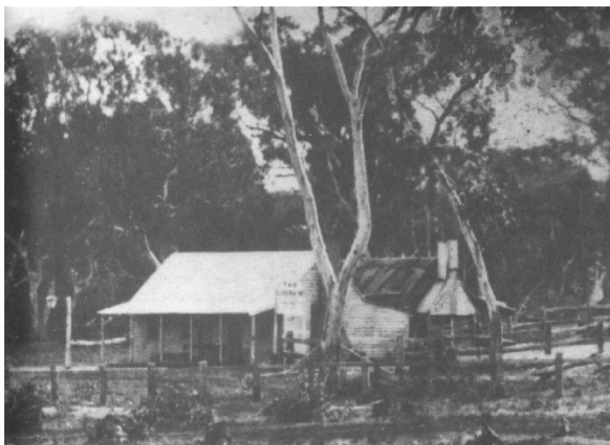
Ann Jones' Glenrowan Inn – “a small unimposing five roomed weatherboard building with a detached slab and bark kitchen at the rear”.
