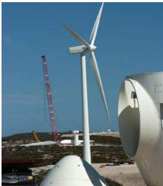
Construction work at Cathedral Rocks Wind Farm
