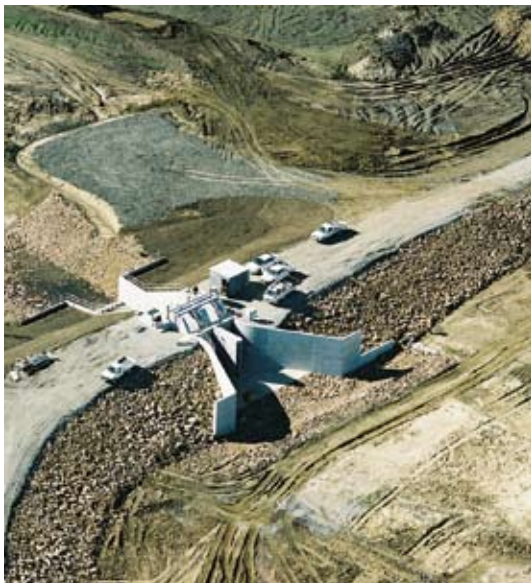
The Poatina re-regulation pond under construction
