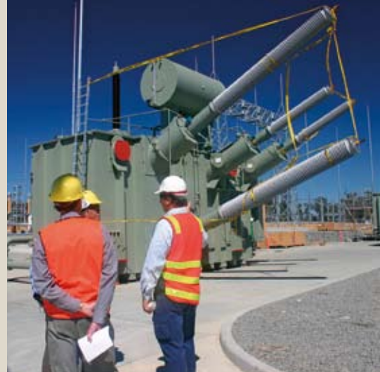
NEM team inspection of Basslink Converter Station at George Town
