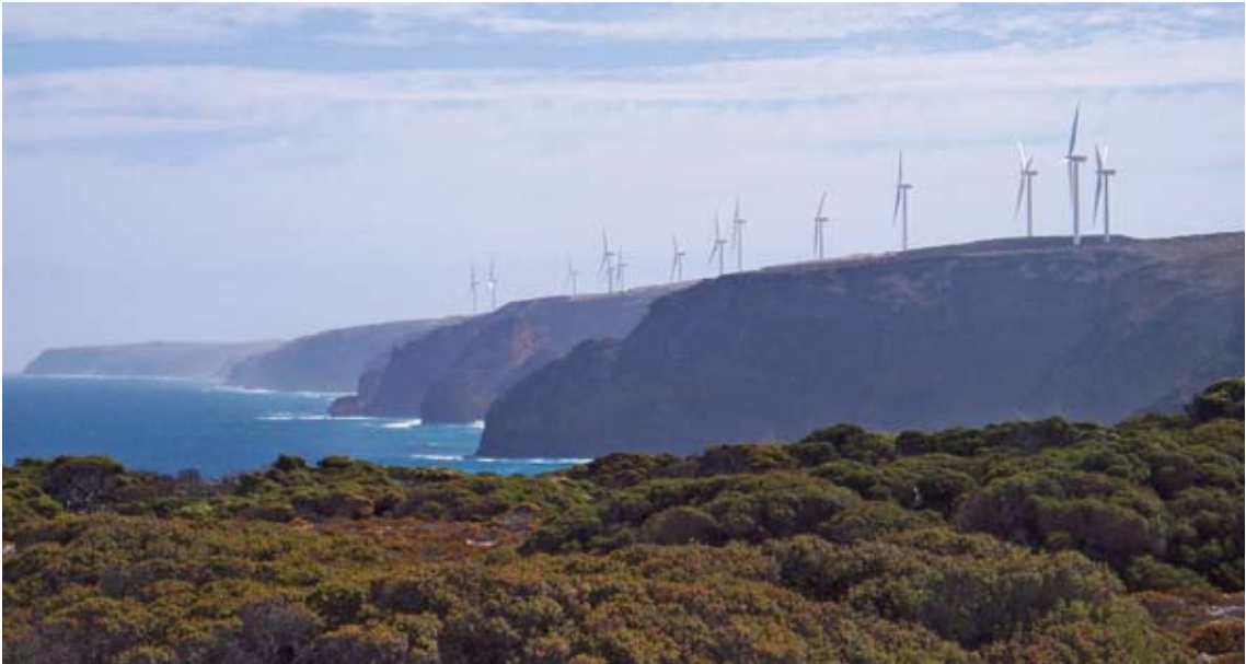
The 66MW Cathedral Rocks Wind Farm in South Australia
