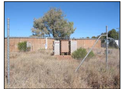
Water Storage Tanks
