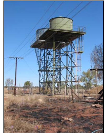
Elevated Water Tanks
