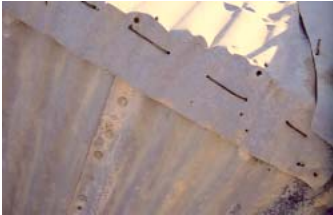
Figure 7.1 Allens Plain Hut ruin chimney showing stitching of corrugated iron – perhaps a pastoralist's, more than a builder's, technique.
