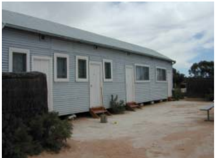
Figure 5.23 Shearers Quarters in 2002 with adaptation visible at far end.
