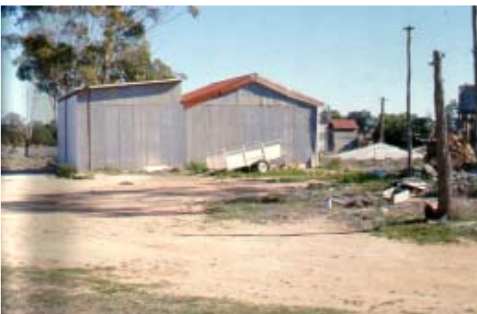
Figure 6.11 Equipment Shed now demolished (NPWS 1986).
