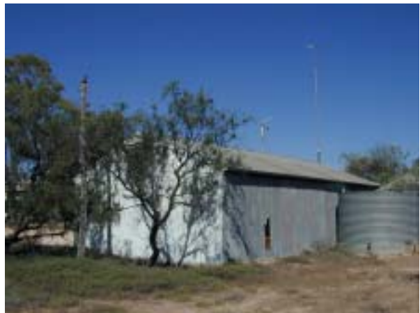
Figure 5.34 Garage constructed c1960.
