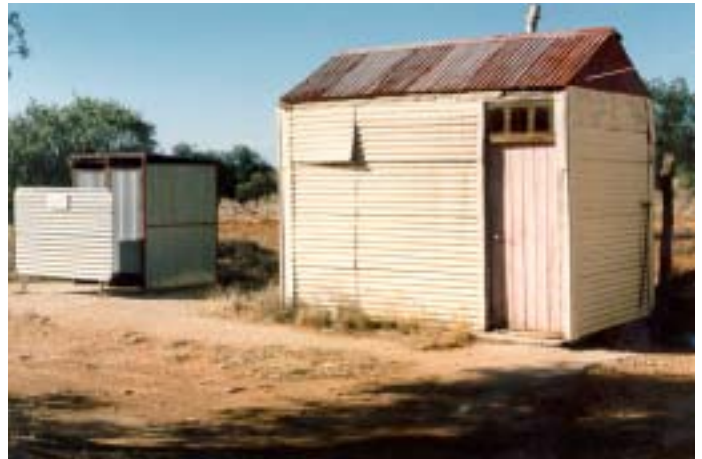
Figure 6.23 Shearers Quarters Bathroom demolished in 1986. Small toilet relocated from Mungo Station by Russell Clothier to the left (NPWS 1986).
