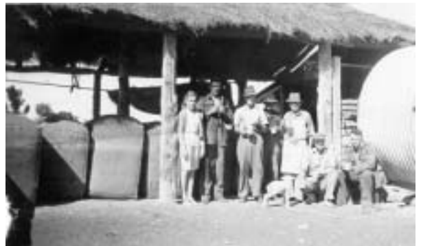
Figure 10.9 The first Woolshed at Zanci, showing post and beam construction with thatch roofing (Barnes family collection).
