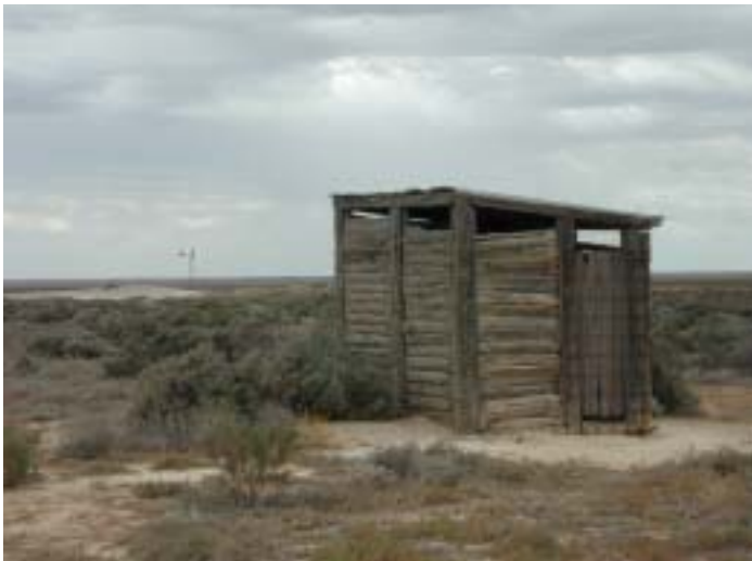
Figure 5.19 'Two-hole' drop-log toilet near the Woolshed that was moved from here from near the Homestead, replacing one that collapsed on this site.
