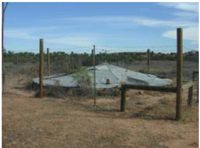
Figure 6.14 Underground concrete tank.
