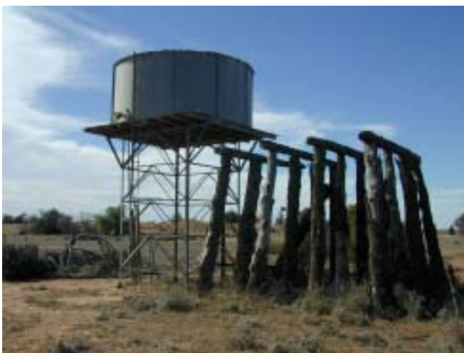
Figure 6.27 Tank Stands near Zanci Homestead area.
