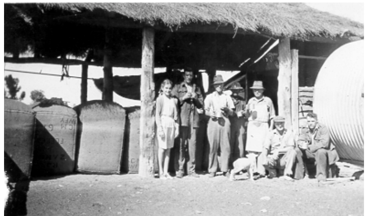
Figure 2.24 The first Woolshed at Zanci, 1949. Notice the open sides with some drop-log construction at the end. Also note the dirt floor and thatched roof. It was replaced by a new Woolshed that reused parts of the Mungo shed. (Appendix D, Image No. 260)
