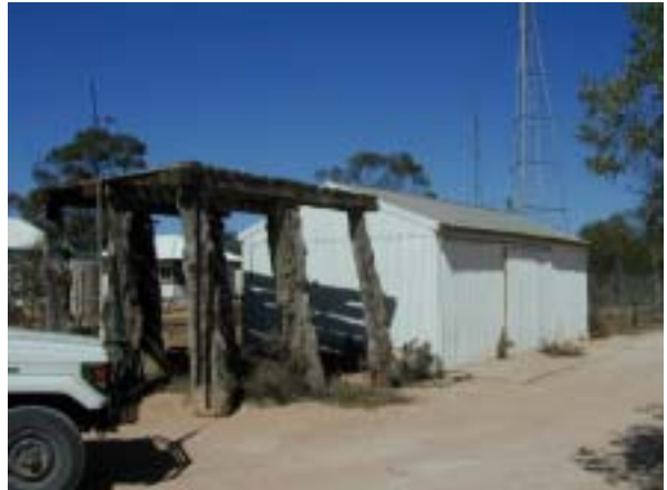
Figure 5.33 Generator shed and pine tank stand. Wind generator tower in the background.
