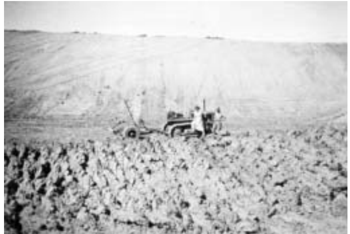
Figure 2.14 Venda and Albert Barnes enlarging the former Scour Tank as the House Tank, 1956. Water was a critical factor in the survival of back-block properties. At Mungo and Zanci numerous tanks were sunk in the landscape to ensure adequate water supply was available. (Appendix D, Image No. 25)
