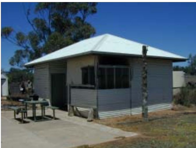
Figure 5.32 Mungo Homestead Laundry on the site of the early drop-log kitchen.
