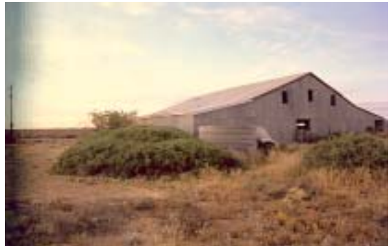
Figure 10.2 Leaghur Woolshed, timber framed with corrugated iron cladding.
