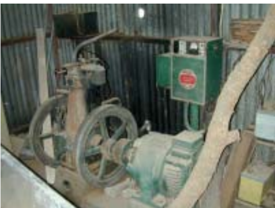
Figure 5.47 Ronaldson and Tippet generator in the Mungo Homestead generator shed.
