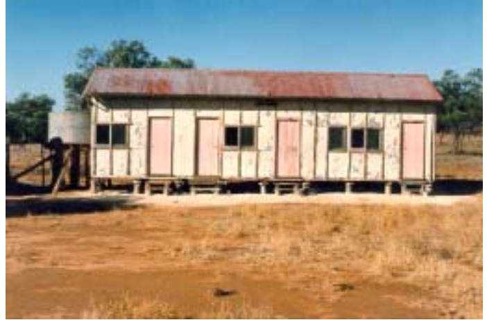
Figure 6.22 Second Shearers Quarters demolished in 1986 (NPWS 1986).
