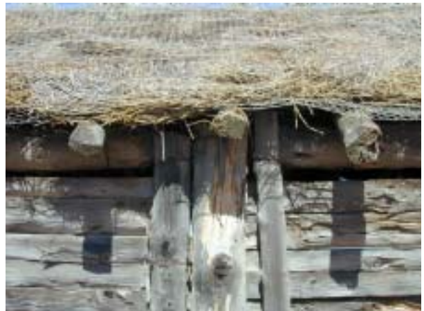
Figure 10.8 Detail of the Zanci stables construction, showing thatch roofing and drop-log construction below. The exterior vertical posts restrain the horizontal timbers.
