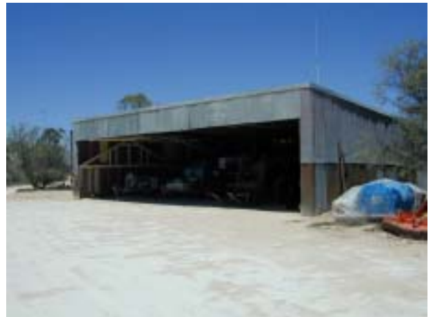
Figure 5.41 Former NPWS Hangar c1982.
