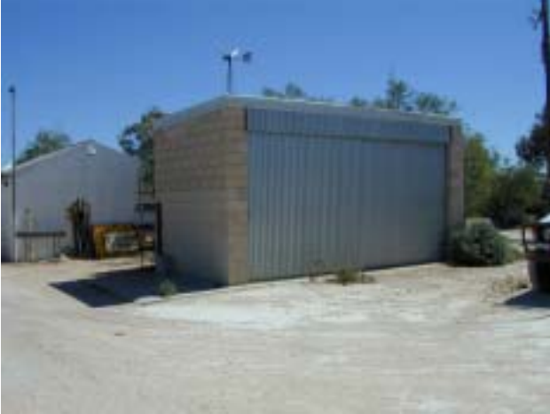
Figure 5.43 NPWS new Generator Shed.
