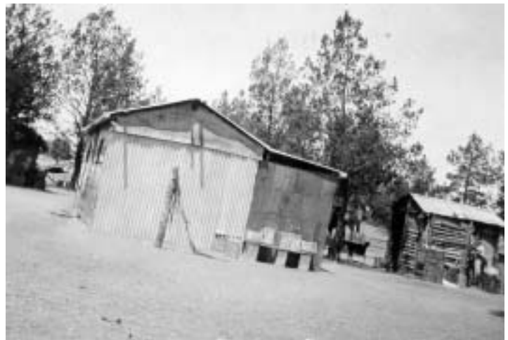
Figure 2.23 The first Zanci Homestead. Built c1925 of flattened kerosene tins and corrugated iron with small drop-log kitchen to the right. This was replaced with a second Homestead. (Appendix D, Image No. 5)
