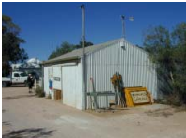
Figure 5.35 Fuel Shed constructed c1960.
