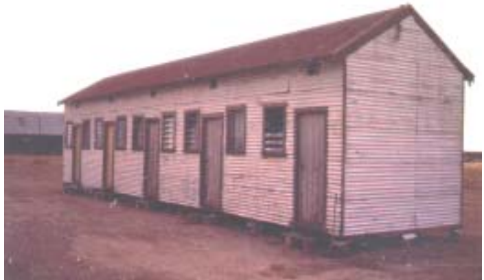
Figure 5.22 Shearers Quarters constructed in 1934 in original form (NPWS photo 1980).
