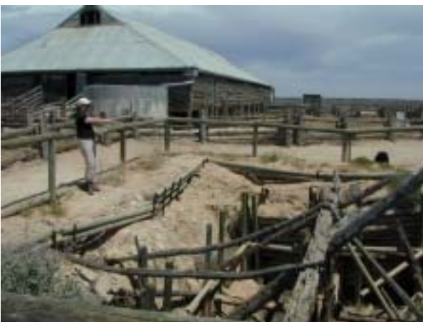
Figure 5.5 The underground logged tank adjacent to Mungo Woolshed
