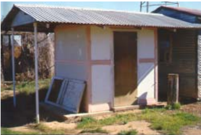
Figure 6.29 Chiller room built near the Second Zanci Homestead by Russell Clothier in the late 1970s (NPWS 1986)
