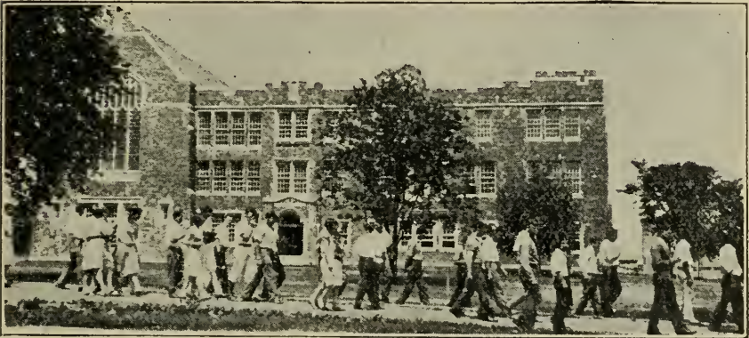
Liberal Arts Building, Blackburn College, Carlinville. This school is unique in that its students are permitted to help pay for their college education by means of the work plan inaugurated seventeen years ago by its president, Dr. William M. Hudson. Of unusual interest to visitors at Blackburn are the Pullman cars used for offices and classrooms.
