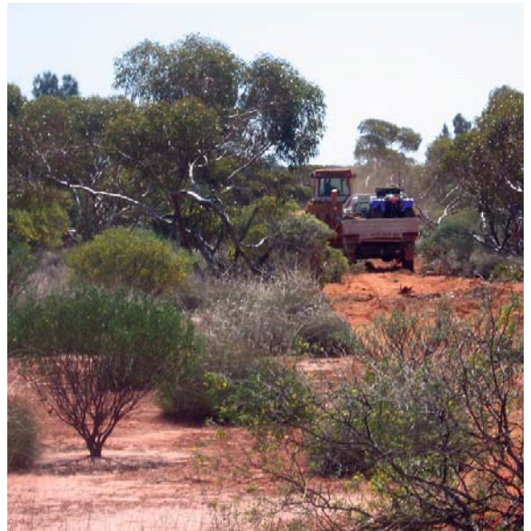
Access track construction. (Photo 406632)
