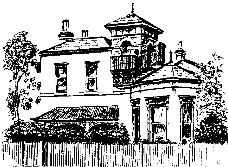
Fig. 6.77 'Doonside', the residence of David Mitchell cnr. Burnley and Doonside Streets (demolished)
