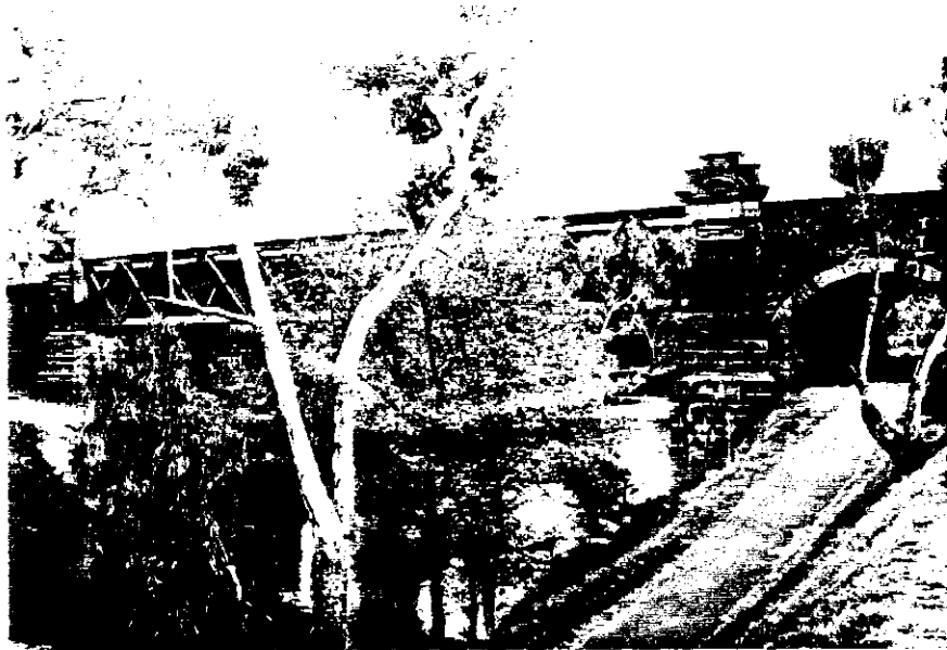
Hawthorn Railway Bridge looking south, 1984.
