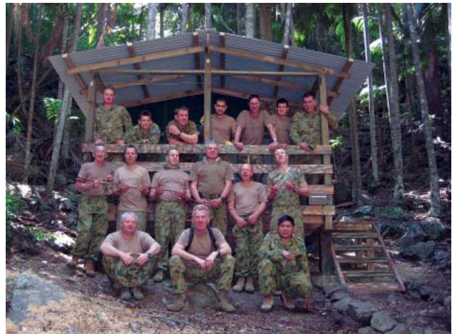
Members from 101st Construction Squadron at the enemy camp where they rebuilt and refurbished a number of structures at the Canungra Military training area during Exercise Jungle Scorpion. Other tasks undertaken included the refurbishment of a 400-metre length of road.
