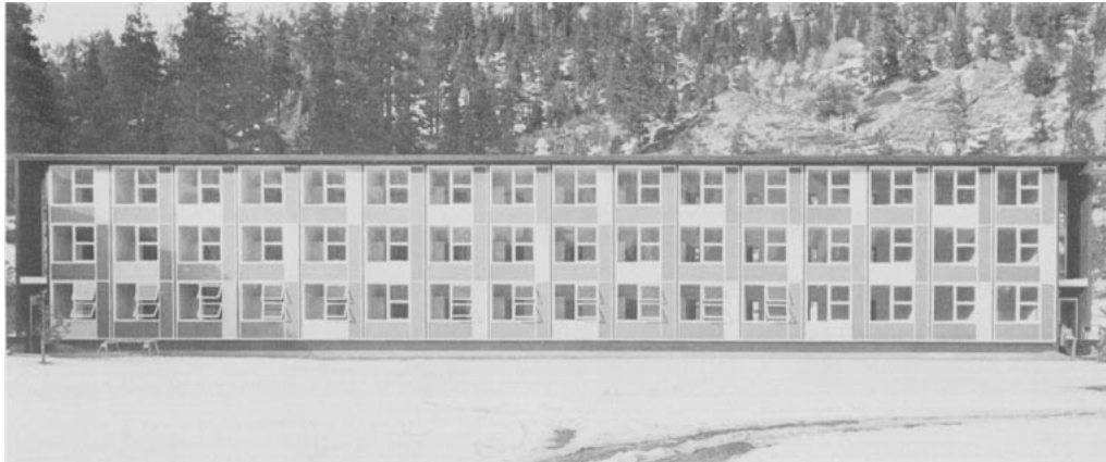
One of the four 75-room Athletes' Dormitories that housed the athletes and team officials in the Olympic Village.
