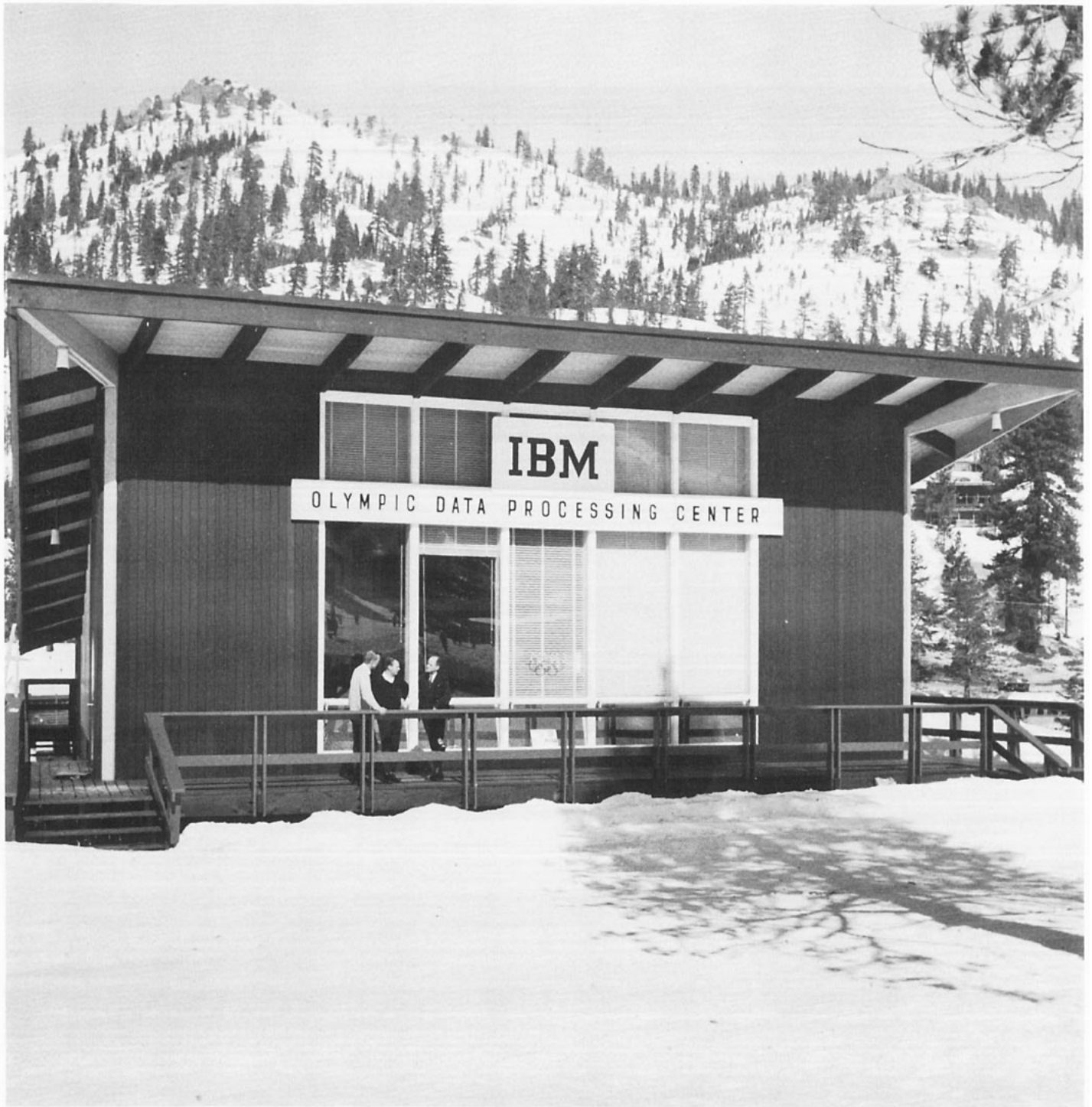
The Olympic Data Processing Center had its own building, in which IBM's 26 volunteers operated the latest in electronic computing equipment. The television broadcasts of the Games also emanated from this building.
