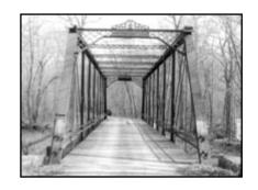
north is an early 20<sup>th</sup>-century metal bridge. Both bridges are Pratt through truss designs. The road linking the two has been identified for its association with early transportation/Underground Railroad.
