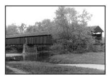
American engineering "combination" bridge form. Bell Ford Bridge, located near Seymour, carried animal and vehicular traffic until 1970 and was used by pedestrians until 1999 when a wind storm damaged half of the span, sending it tumbling into the White River. Local officials have retrieved heavy timbers and metal fittings to reconstruct this span of the two-span bridge.
