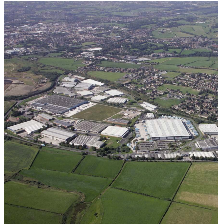
Heywood Distribution Park, UK
