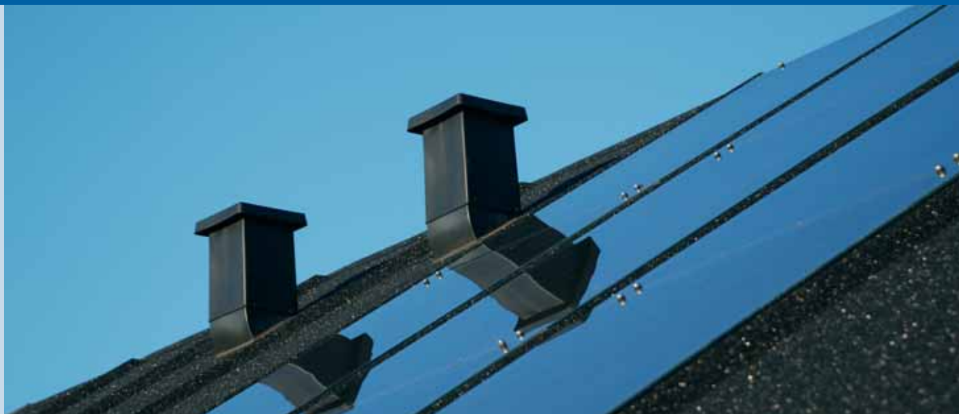
Fig. 1 - Reflections in the dark modules which are customized to be a natural part of the roof in colour and shape.
