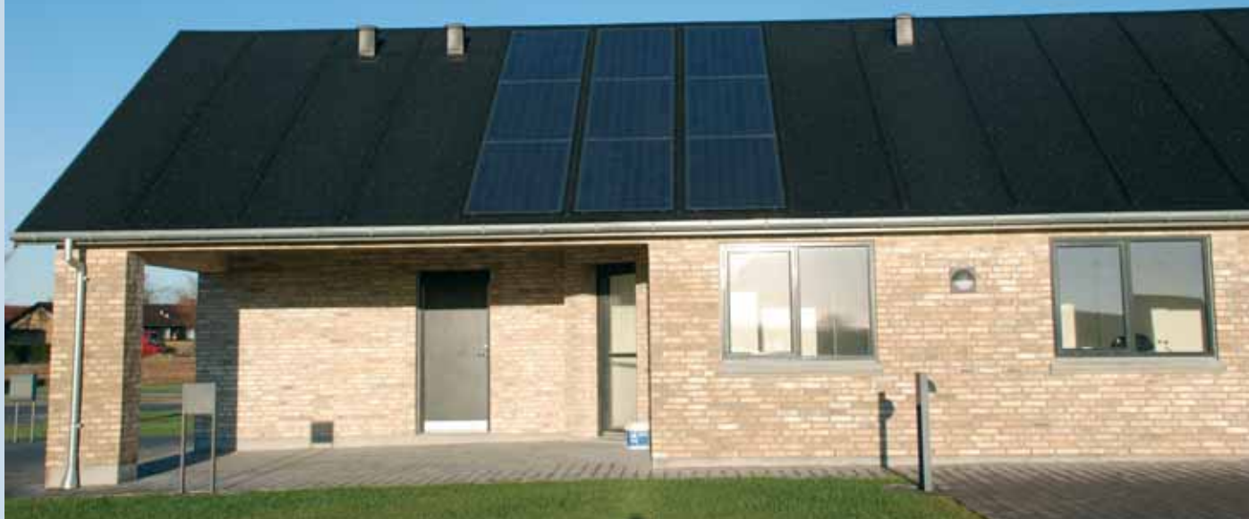
Fig. 2 - The customized PV modules from the Danish module manufacturer GAIA Solar are made especially to fit with the roof in the PV-Danmark project.
