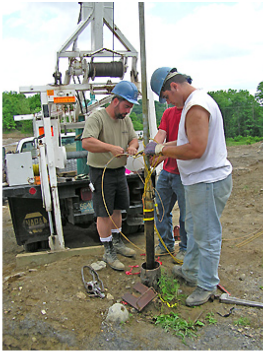
Figure 2. DEP fields crew installing a packer. Photo by L.J. Nicholson
