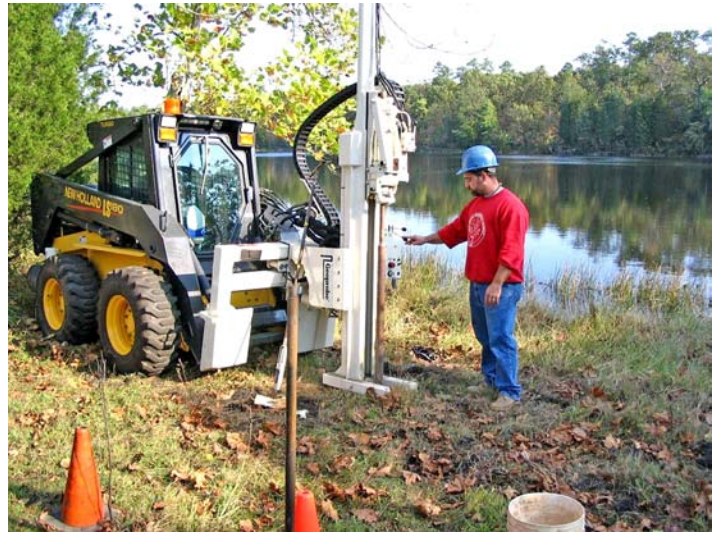
Figure 3. Greg Steidl used the geoprobe to collect a soil core. Photo by S.W. Johnson
