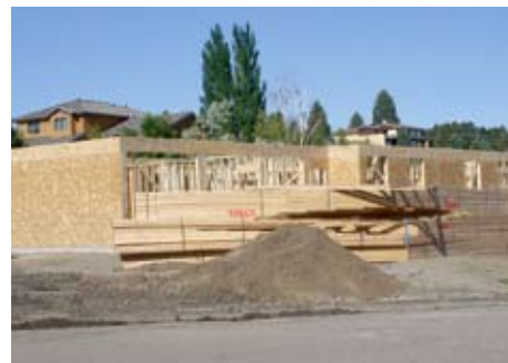
Quality topsoil is the basis for quality landscapes.
