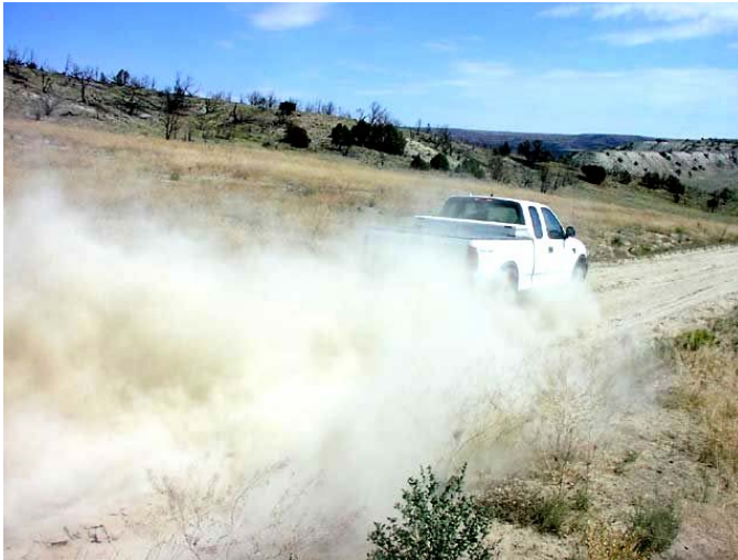
Figure 1. Photo (1) . Dust typical of untreated roadway.
