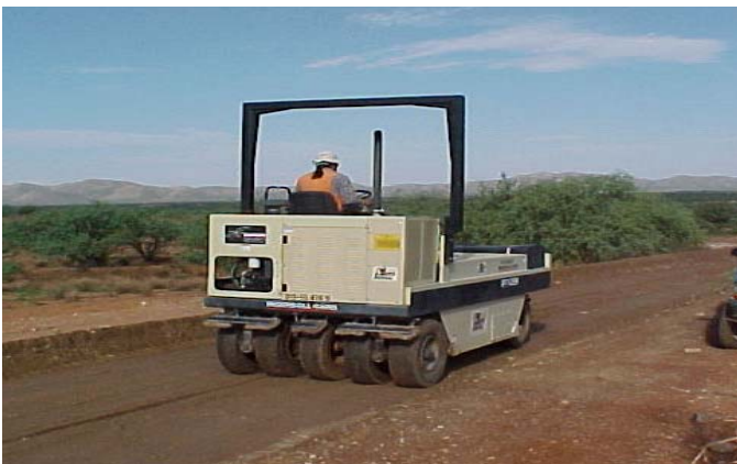
Figure 7. Photo. Typical rolling and compaction.
