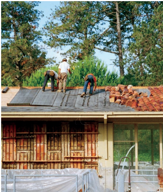
Workers replace the wooden roof at Upper San Leandro and add a plywood diaphragm over diagonal timber sheathing to provide additional strength to the building.
