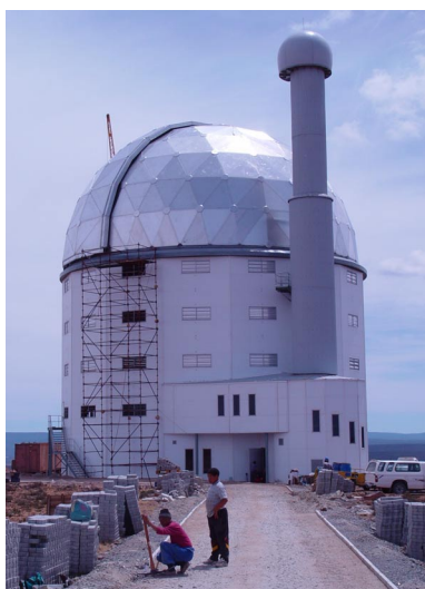
Fig.6. SALT under construction in Sutherland.
