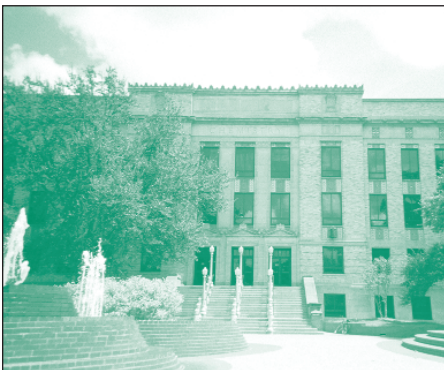
Chemistry Building (Texas A&M University)
