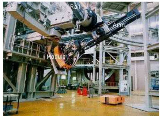
Figure 23 - Blanket Maintenance Facility
