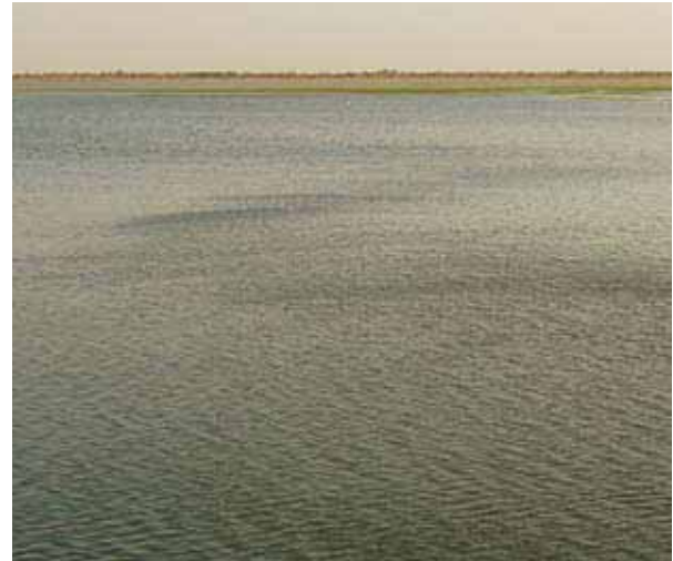
Islands and seasonal grasses are visible in the Sennar dam reservoir, which is now 60 percent full of sediment
