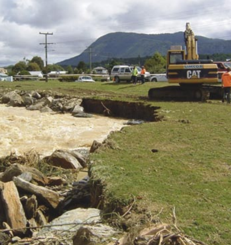
Repairs to Waikawa Stream bank
