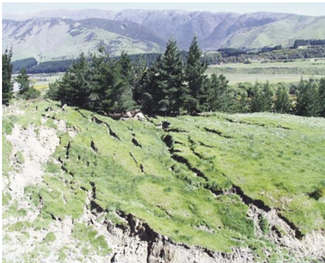
Large landslide - Awatere Valley
