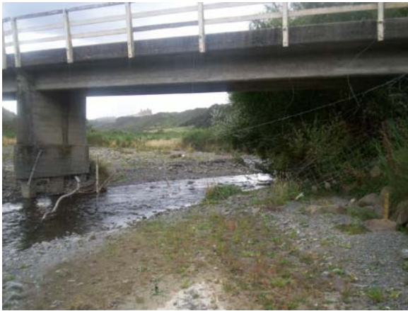
Figure 11 - Charwell River at Stag and Spey Rd Bridge
