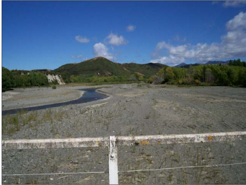
Figure 6 - Ferniehurst Bridge looking upstream, November 2006.
