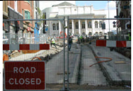
Work in progress on Nottingham's new tram system
