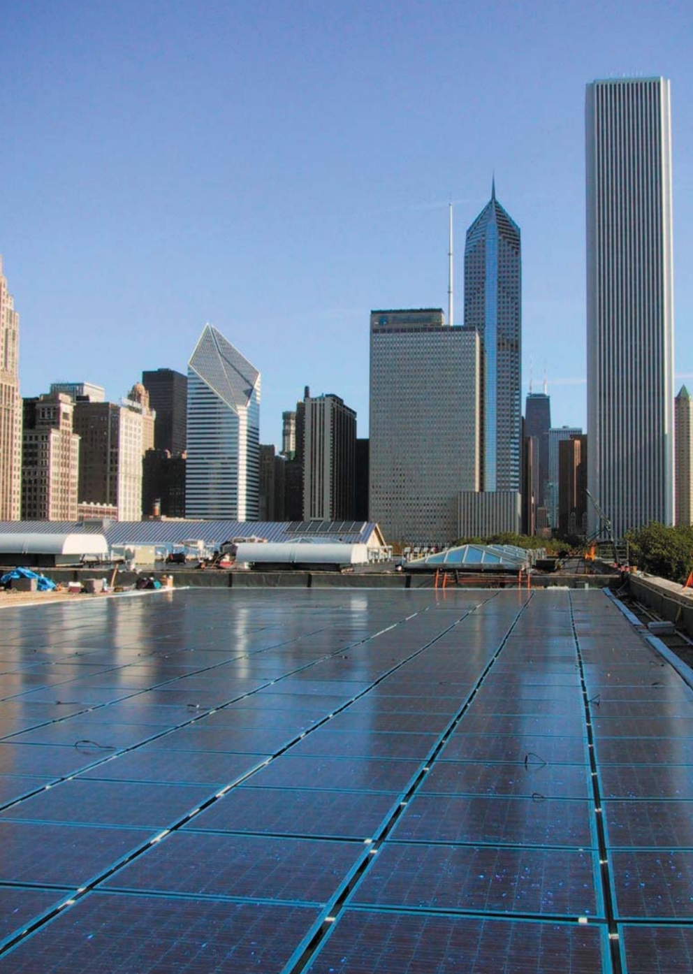
Spire Solar Chicago, NREL PIX 13789
