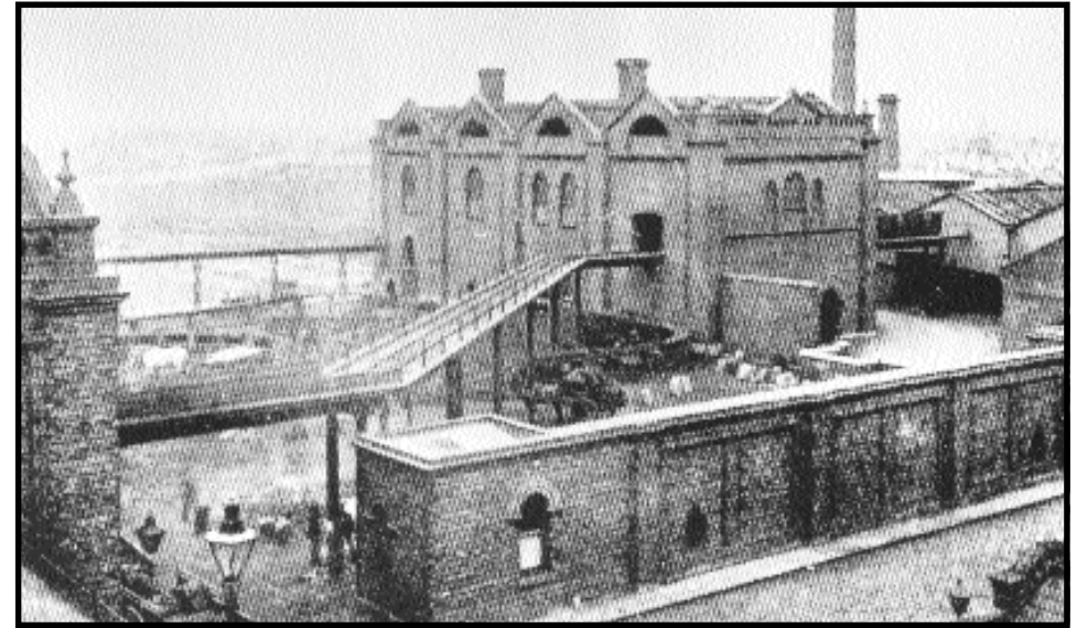
The former Gasworks, now Gasworks Park
