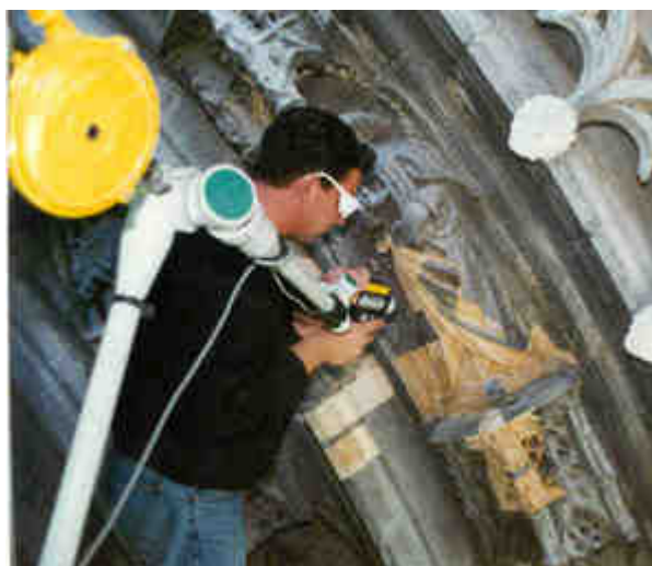
Photo 2: Test of laser cleaning on a sculpted arch stone as part of the preliminary study for the restoration of the north portal of the Saint-Michel Basilica in Bordeaux (Photo: T. Vieweger).
