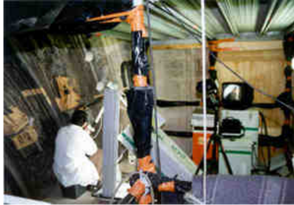
Photo 4: Interior of work zone on a laser cleaning site (restoration of the north portal of the Saint-Michel Basilica in Bordeaux (Photo: T. Vieweger).
