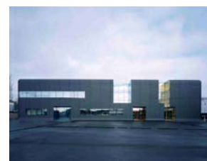
Centre bus de Thiais
