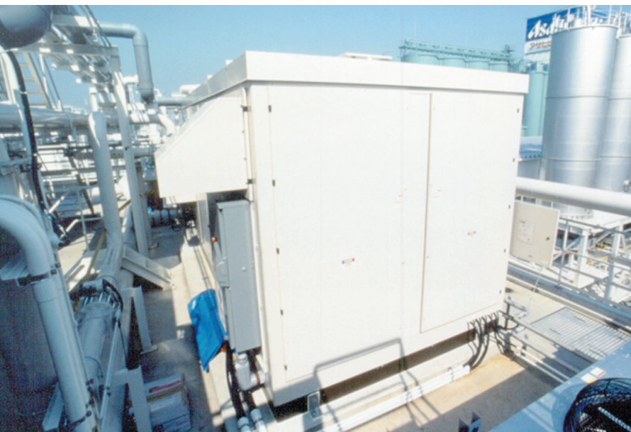
Photo 1. This fuel cell produces electricity using hydrogen from the waste gases of the brewing process at Asahi Brewery in Japan.
