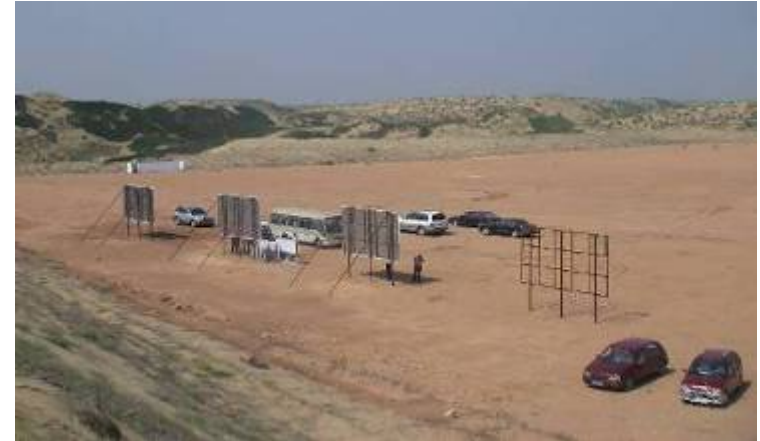
Shaanxi: selected CTL site with initial ground works done
