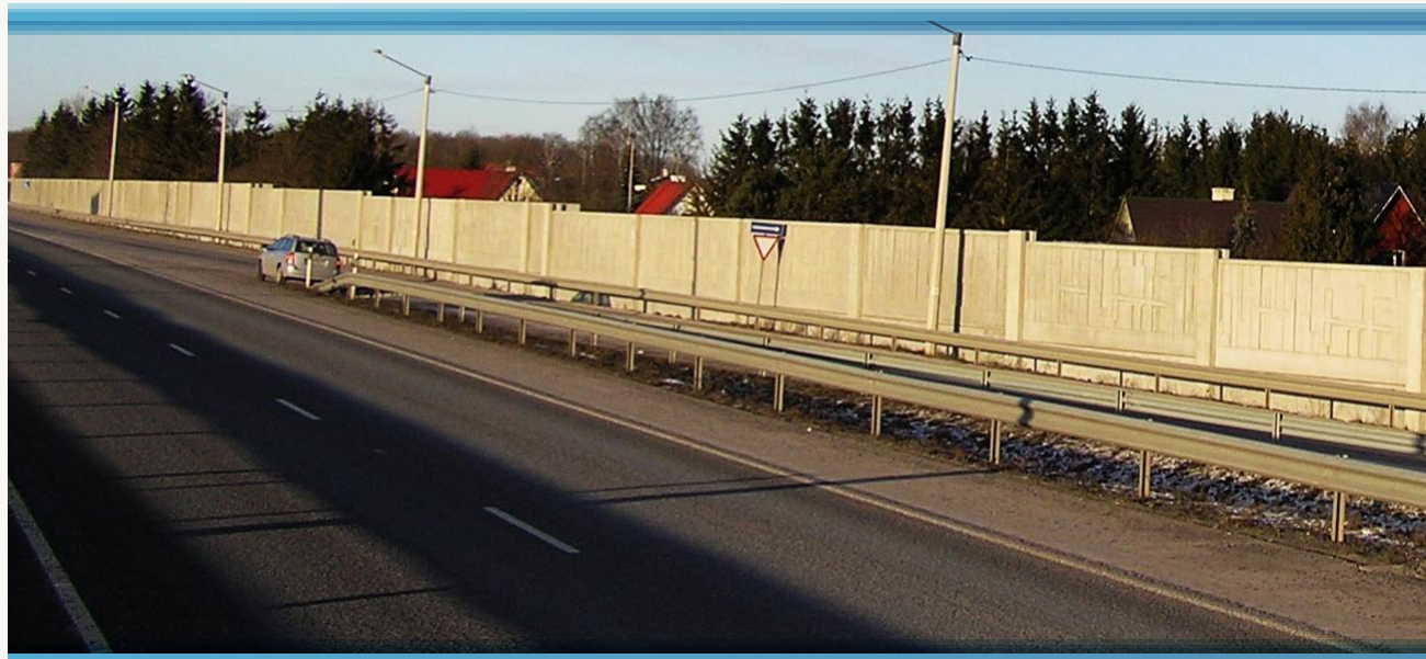
The Pildiküla noise barrier wall, completed in 2007.
