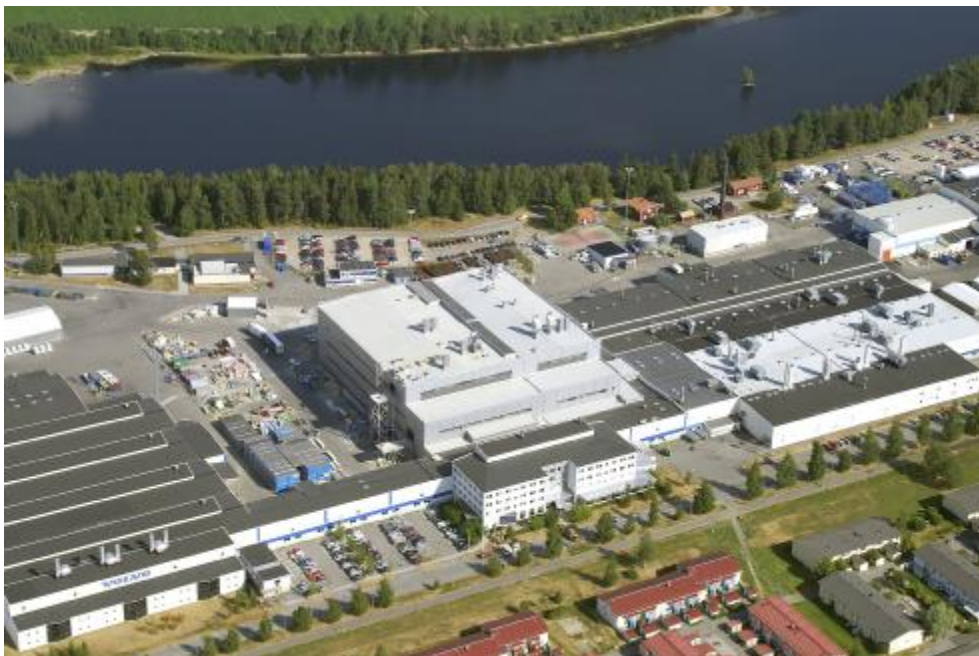
The new topcoat paint shop at Volvo Trucks in Umeå, Sweden, is an advanced and fully automated facility.
