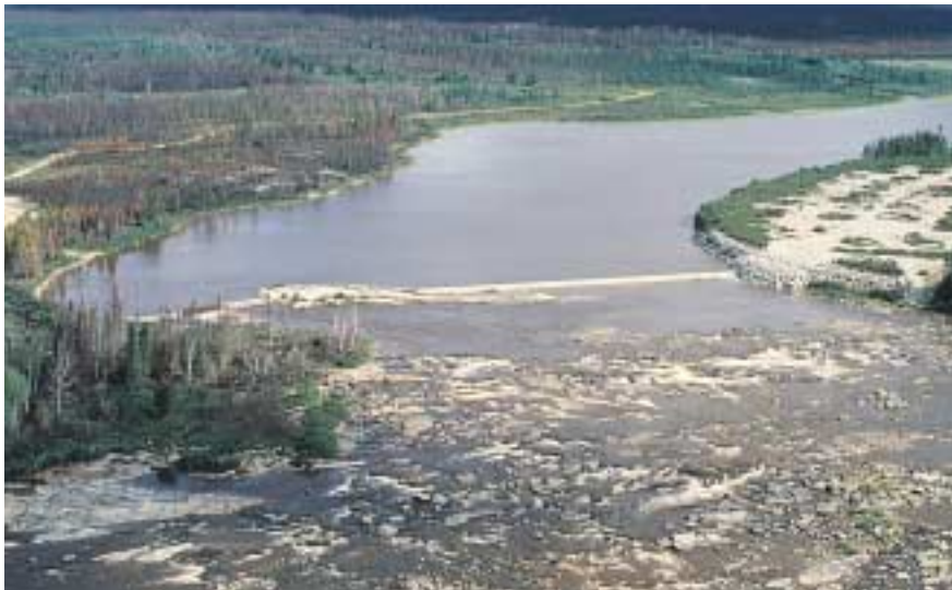
Weir no. 8 on the Opinaca River. Note planting on the right, and traces of a recent fire on the left.
