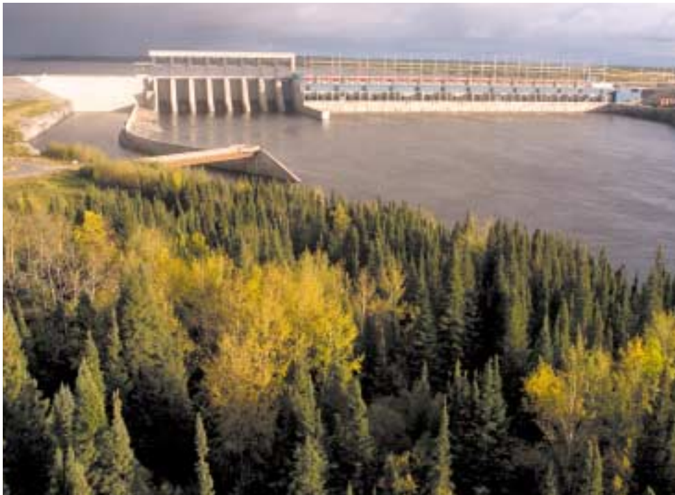
La Grande-1 hydroelectric development, viewed from downstream.
