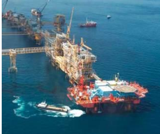
Figure 4: Oil production facility
