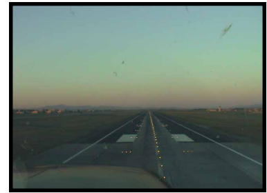
Completed runway and lighting project at Fairchild AFB
