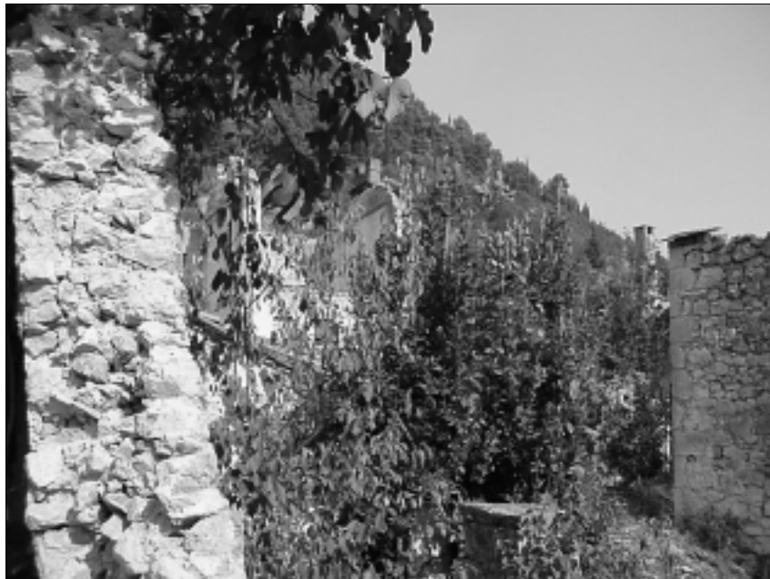
Hatid'a Behmen's house after its destruction (July 1993)
