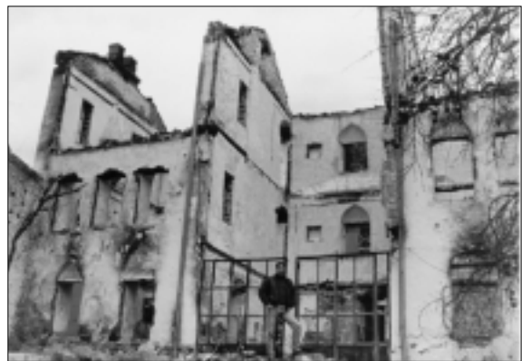
The house of Had`i-Salih Behmen after its destruction in July 1993
