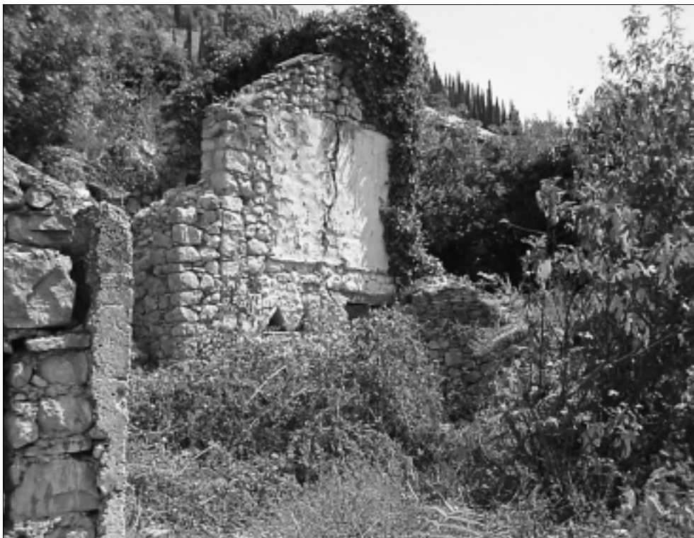
The Repkovina housing complex in Uzinovi}i after its destruction (July 1993)
