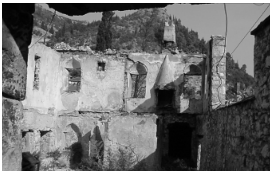
@uja's house after its destruction (July 1993)
