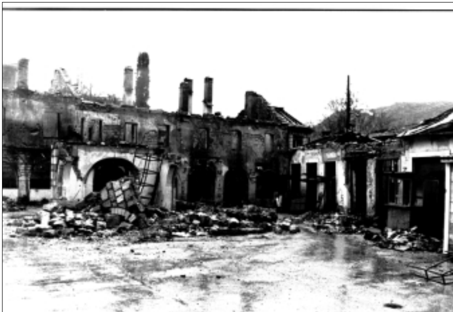
Silahdar Husein-pa{a}'s Lodge in Tepe , after its destruction in July 1993
