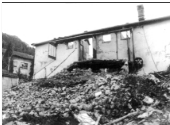
The houses of Ivo Babi} and Avdo Trklja. The former burned, the latter dynamited.
