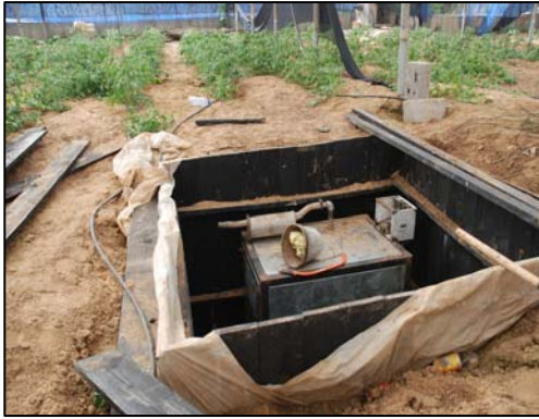
Generator and digging equipment near the tunnel shaft. The generator was sunk into the ground to muffle noise and make its discovery difficult (IDF Spokesman's Website, August 16).
