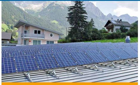
A 26,7 kW grid-connected system on a flat roof in Anterselva, Bolzano, Italy.
