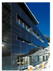
A private home in St. Moritz, Switzerland. The integrated energy concept incorporates a 22,5 kW structurally glazed PV façade, solar thermal collectors and a heat pump. [PHOTO/ARCHITECT JOSEF TROXLER]
