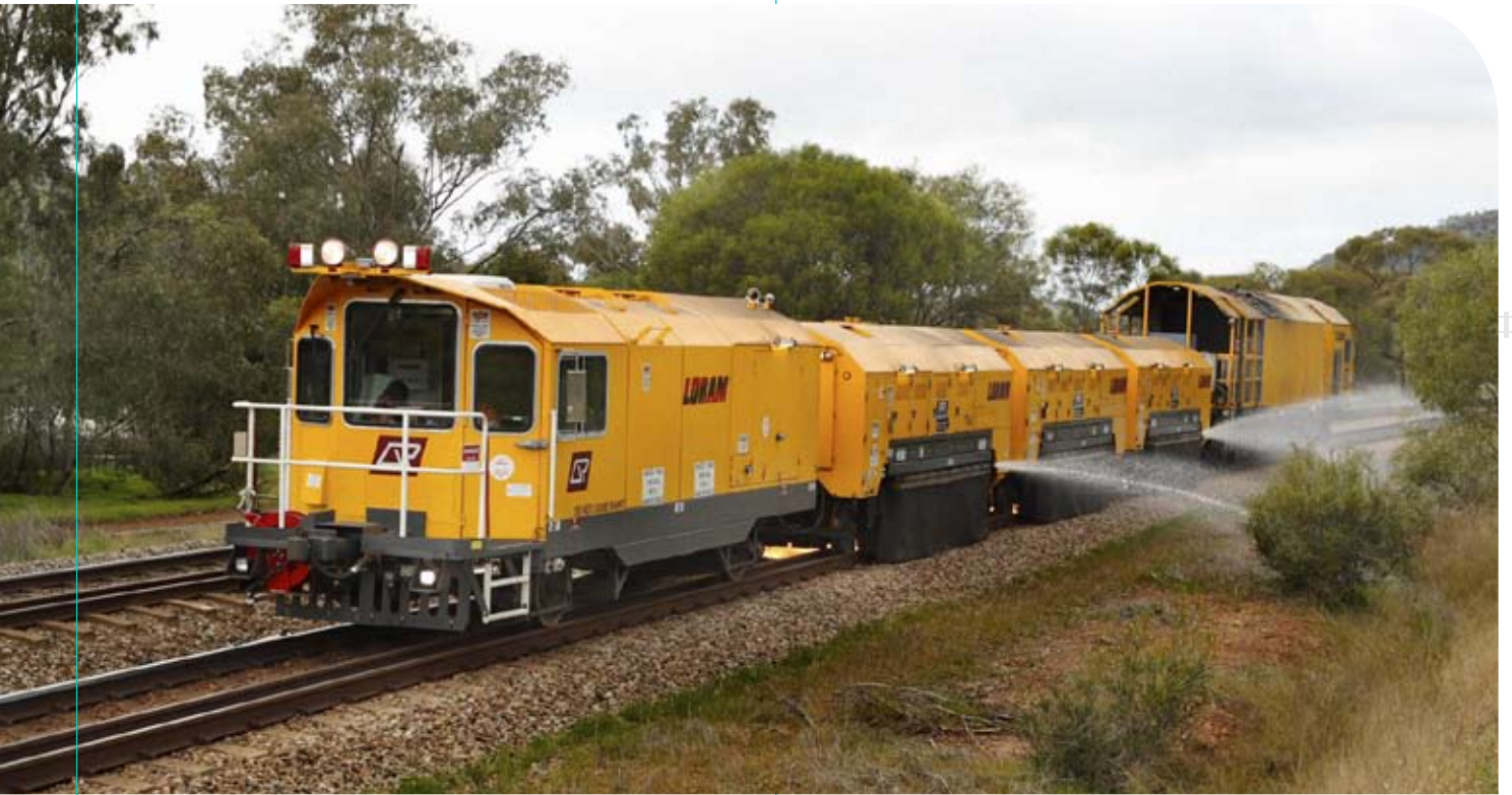
QR's new rail grinding service in operation in Western Australia.
