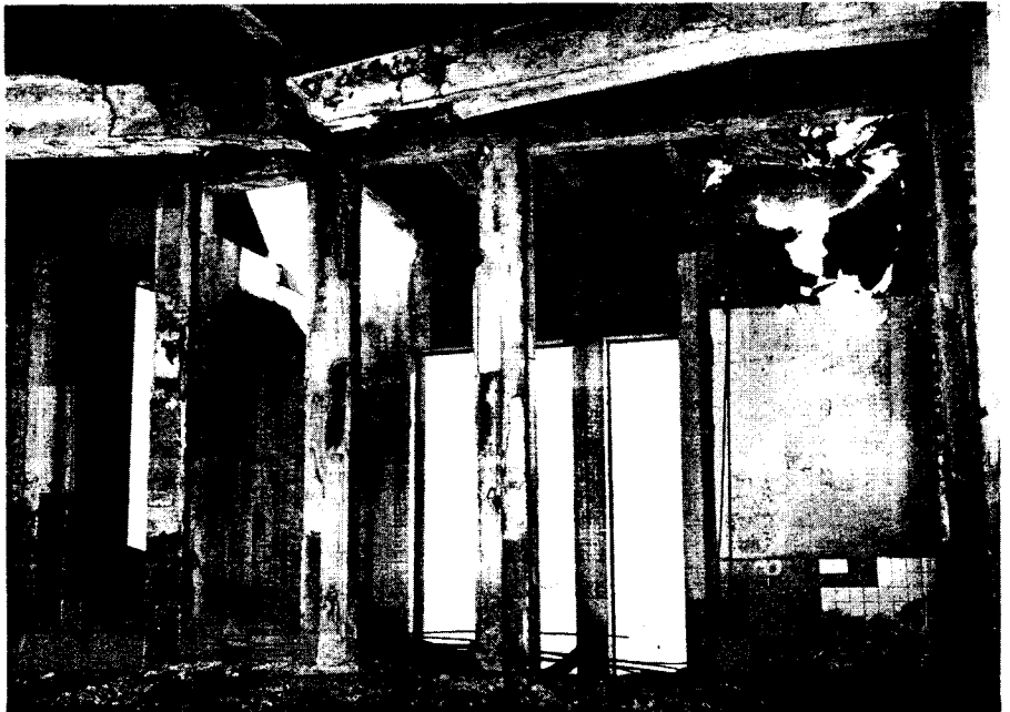
Figure 5.20a. Upper photo: Reinforced-concrete, aseismic structure; window fire shutters were blown in by blast and the interior gutted by fire (0.12 mile from ground zero at Hiroshima). Lower photo: Burned out interior of similar structure.
