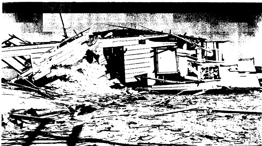
Figure 5.70. Rambler-type house after a nuclear explosion (5 psi peak overpressure).
