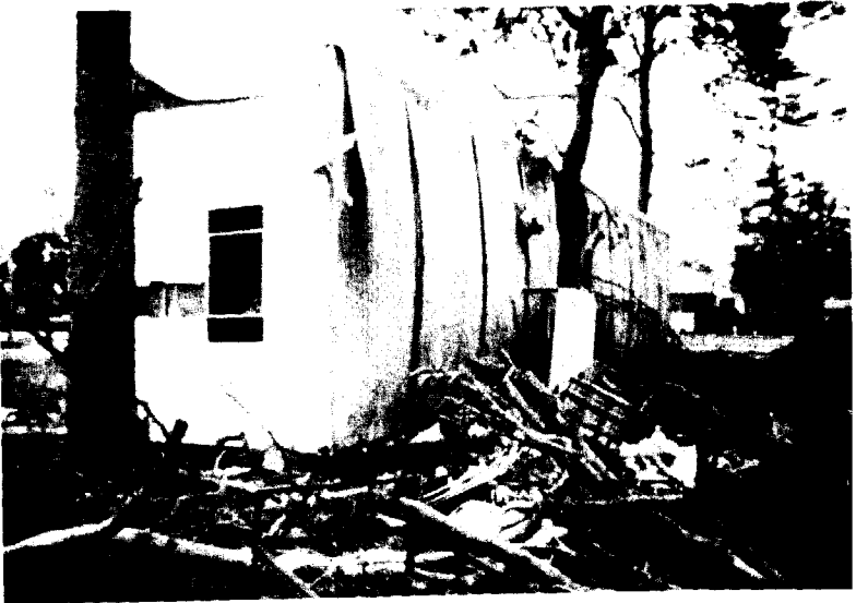
Figure 17a (top) and 17b. Hurricane Kate (1985) damage (From Clark, 1986b).
