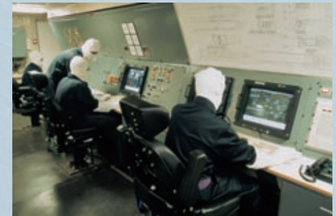
Machinery Control Room
