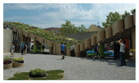
team eventually chose to apply a dual layer of recyclable plastic waterproofing, as well as layers of lacquer and polyurethane coating on the tube surfaces.
