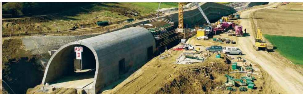
Tullnerfeld section of Westbahn route – Hakenfeld tunnel
