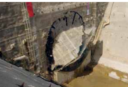
Through-cut of Stierschweiffeld tunnel
