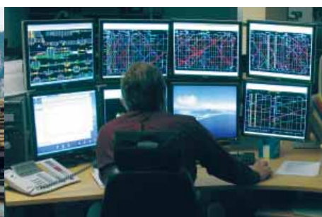
Traffic control center
