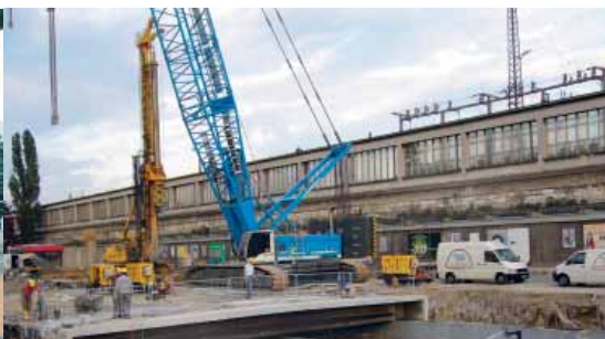
Main railway station Vienna – construction work on forecourt Südtiroler Platz
