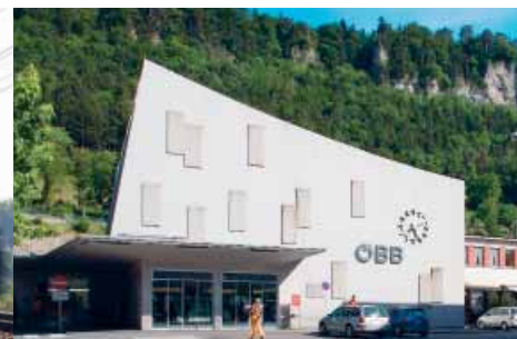
New railway station Feldkirch
