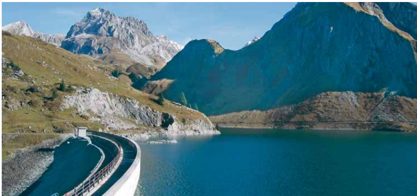
Spullersee, storing reservoir of the power plant
