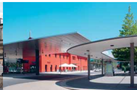
New railway station Feldkirch
