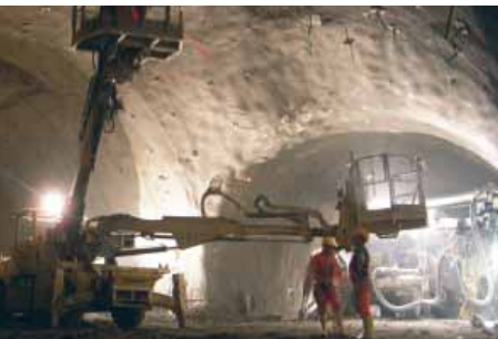
Driving of Wienerwaldtunnel
