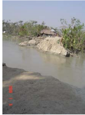
Photo 3.20. Failure of the local embankment due to excessive water storage gathered from storm surge
