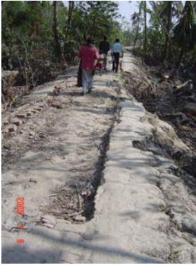
Photo 3.19. Damaged local road
