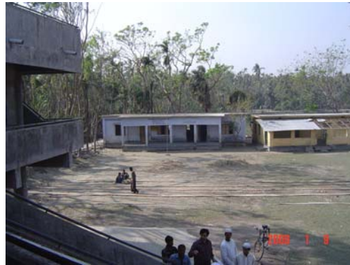
Photo 3.8. Primary school and mosque of the multipurpose cyclone center
