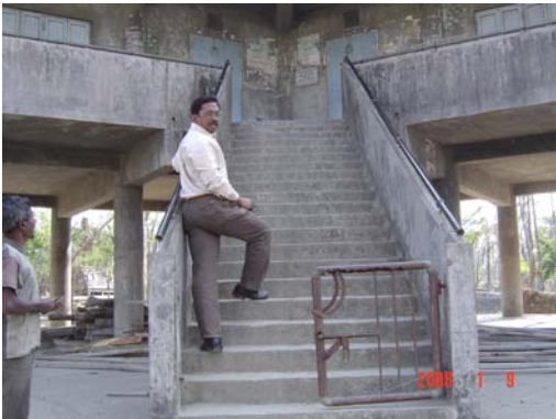
Photo 3.9. Surge water level was about 8 steps of the stairs shown by local people
