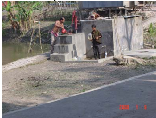
Photo 3.12. Water supply of the shelter is mainly by hand tube-well
