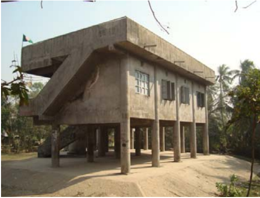
Photo 3.1. Cyclone center Kanainagar where no storm surge occurred
