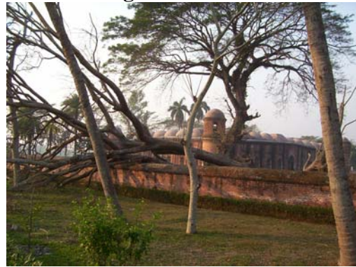
Photo 3.30. Heritage site “Sat Gombuj Mosque” is narrowly escaped from a fallen tree.
