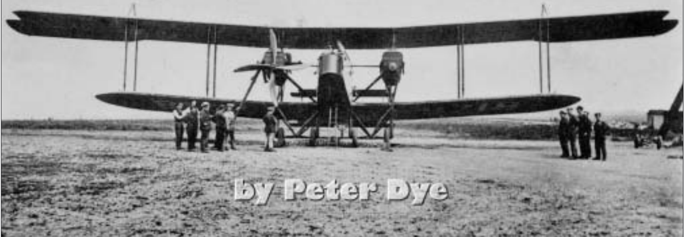
Handley Page O/400, C or D9718 of No 58 TDS at Cranwell in 1918, showing the size of the bomber to good effect. With an endurance of eight hours and a top speed of 97.5 mph (at sea level) it was ideally suited for the proposed flight to Egypt. :RAF College Library
