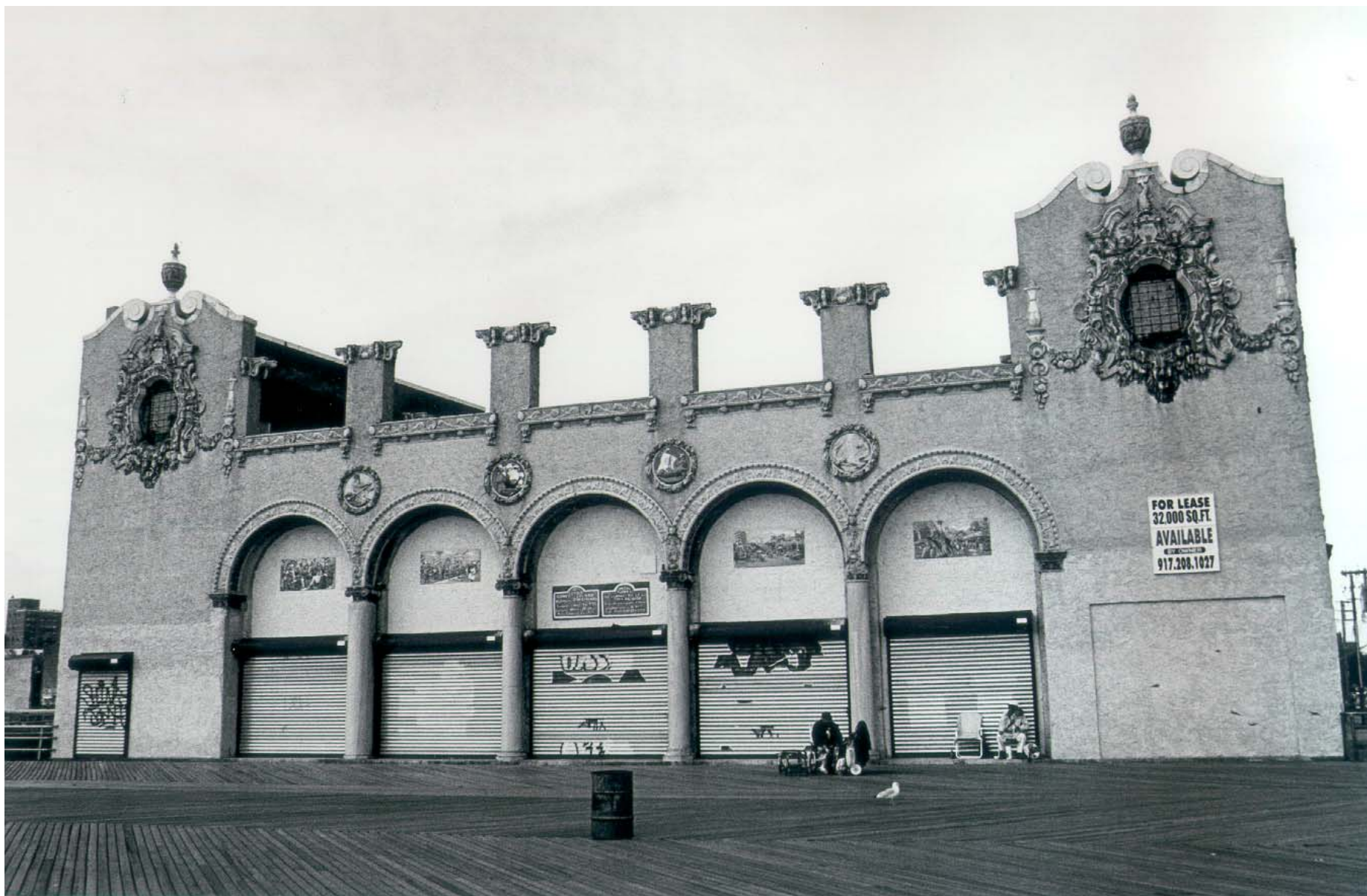
(Former) Childs Restaurant Building 2102 Boardwalk (aka 3052-3078 West 21 st Street), Brooklyn Photo: Carl Forster
